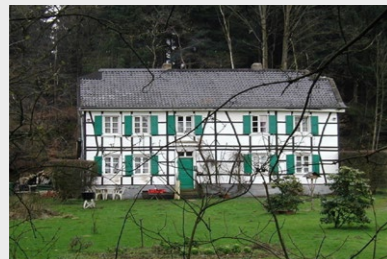
Pulvermühle Aue, Foto LuGev
